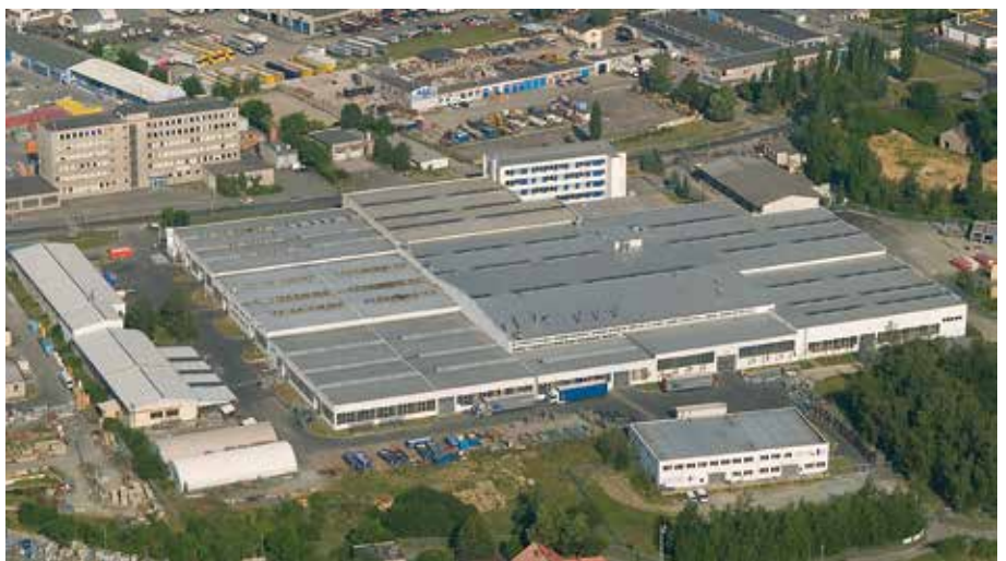
Production site in Pilzen (CZ) with over 29.082 m 2 roofed production space
